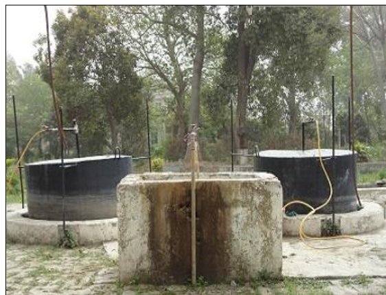
Figure 3: Formation of biogas in control and experimental digesters. The right being control and the left served as the experimental digester.
