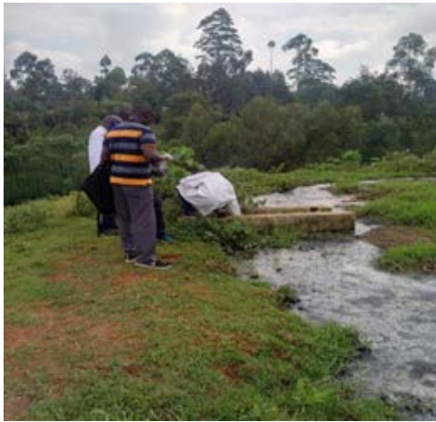
Plate 6: Savona Lagoon Overflowing
