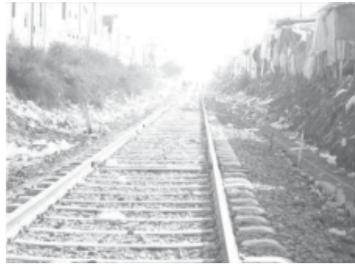
Figure 3: Dumping of communal waste on Railway line
