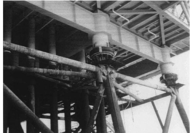
Figure 5: Photograph showing seismic isolators at the top of the jacket
