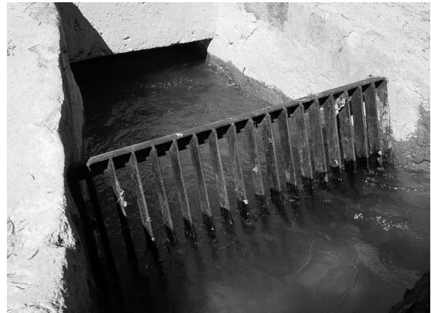
Figure 3: Placement of trash rack
