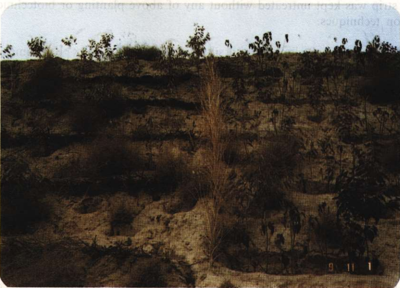
Fig. 4. Photograph showing staggered contour trenches on right side plot and brush layering on left.
