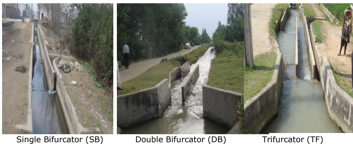
Fig. 2: Types of crump weir
